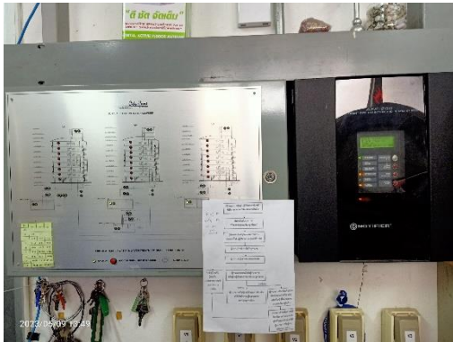
Fire Alarm Control Panel : FCP
